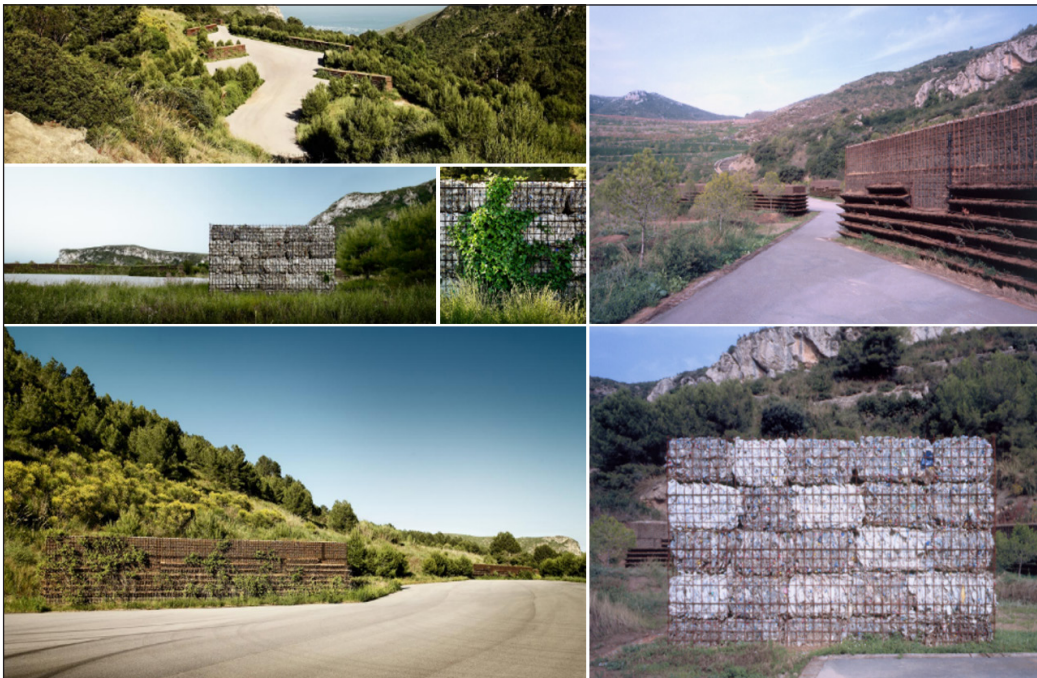
Figure 4. Landscape features made by waste materials to keep the history of the site and educational purposes in the Vall d'en Joan landfill site, Spain (Batlle & Joan Roig, 2011)
